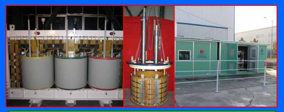
The 630kVA/10.5kV/0.4kV HTS power transformer was installed at the headquarters of TBEA in Changji City, Xinjiang Autonomous Region, and was energized on November 21, 2005.
